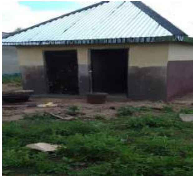
Pic. 2: Construction of two modern squatting toilets at RCM Primary School, Ijege.
